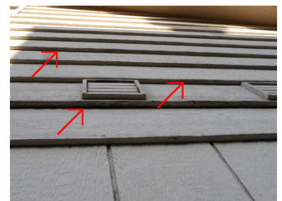
Siding is water damaged/checking
