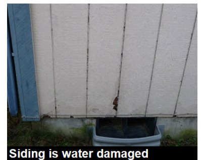
Siding is water damaged/checking
